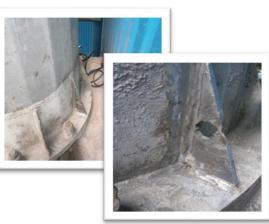
The solution: The concrete surrounding the defective fixing of the mast was first broken out, in order to facilitate the Ancon coupler and new bolt, which were installed and tightened to the required tension. Existing concrete surfaces were primed, and new concrete was instated to
