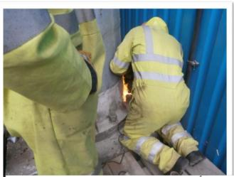
form the original concrete profile, before a new stiffener plate was welded to the corroded stiffener. existing Upon completion, the exposed steel was coated to provide additional weather protection.
